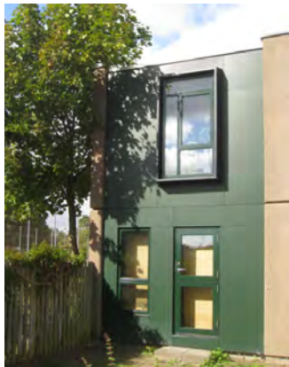
Galgebakken mock-up af facade november 2014 og september 2015
