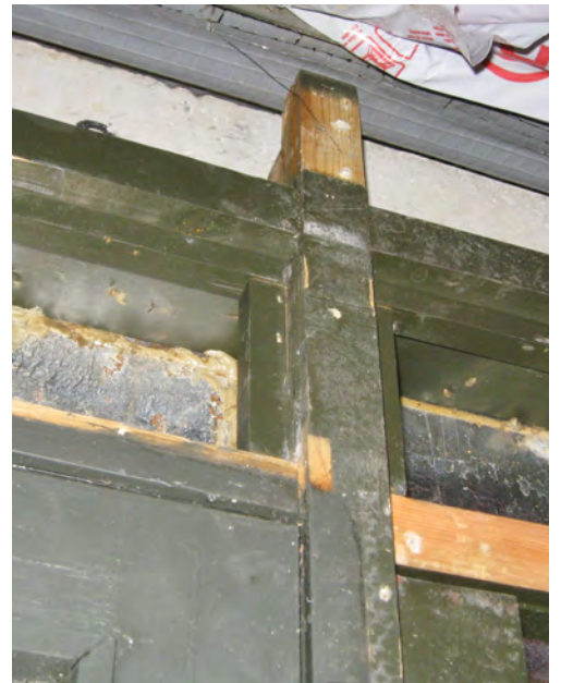
Galgebakken mock-up af facade 18. november 2014
