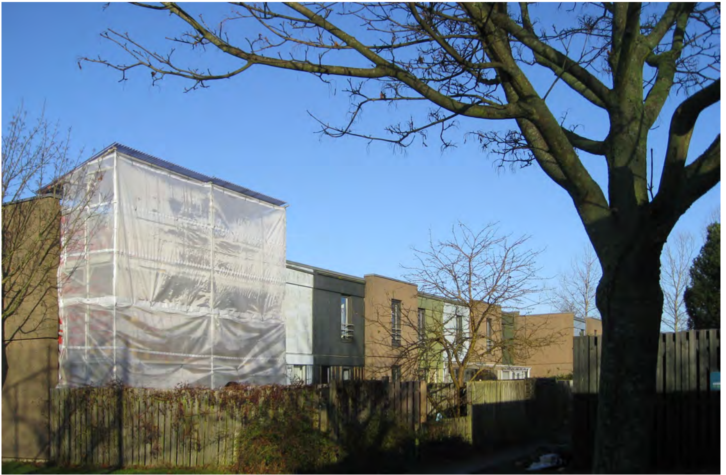
Galgebakken mock-up af facade 25. november 2014
